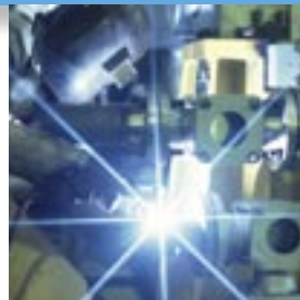
Weld seam testing
